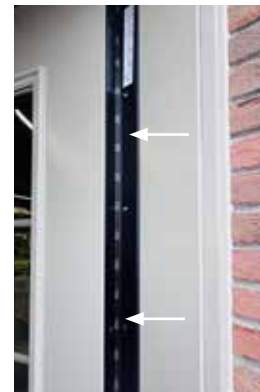
CONTINUOUS HINGE - OPEN
