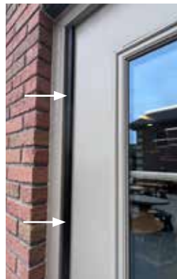
CONTINUOUS HINGE - CLOSED
